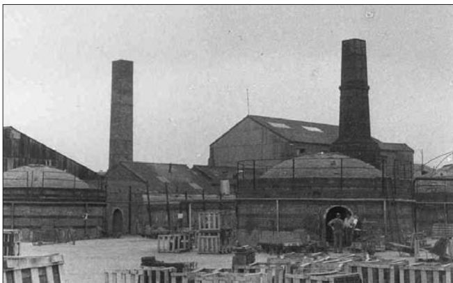
Keymer Works showing two "Beehive Kilns" with domed roofs, c. 1980 (Fred Avery)
