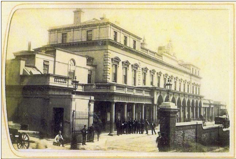
1840 Brighton Station building in it's early form (Charman Family collection - Southwater Local History Group)
