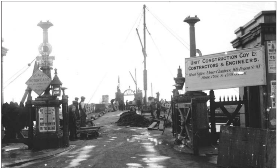
Stage in demolition of original, 1833, bridge, note the clutter of signs at the eastern gateway (by kind permission Marlipins Museum, SAS)
