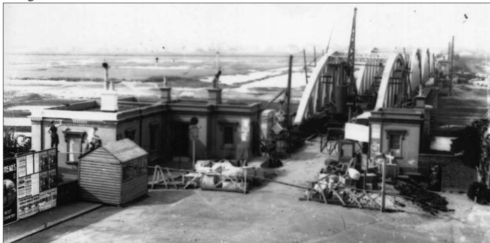
Taken during later stages of building the 1923 Norfolk Bridge, shows at left the three stages of construction of the toll house can be seen (by kind permission Marlipins Museum, SAS)
