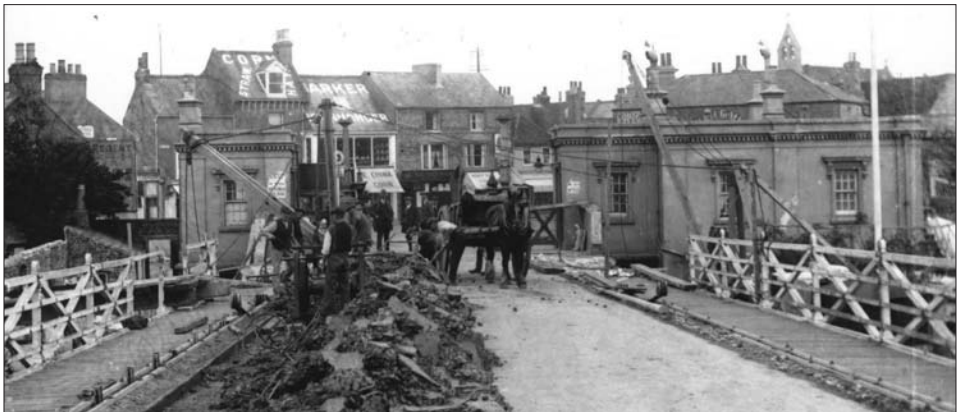
Taken during demolition of the 1833 Norfolk Bridge, shows at right the original and second stage of construction of the toll house (by kind permission Marlipins Museum, SAS)
