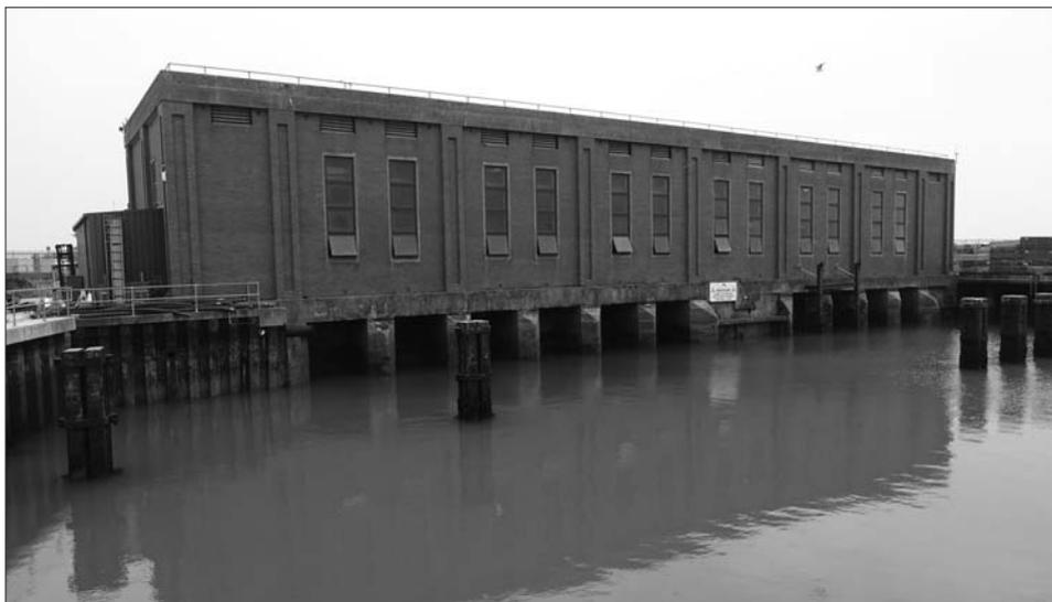
The combined pump house for the cooling water for the electricity power station and to maintain the water level in the harbour arm at Shoreham Harbour.
