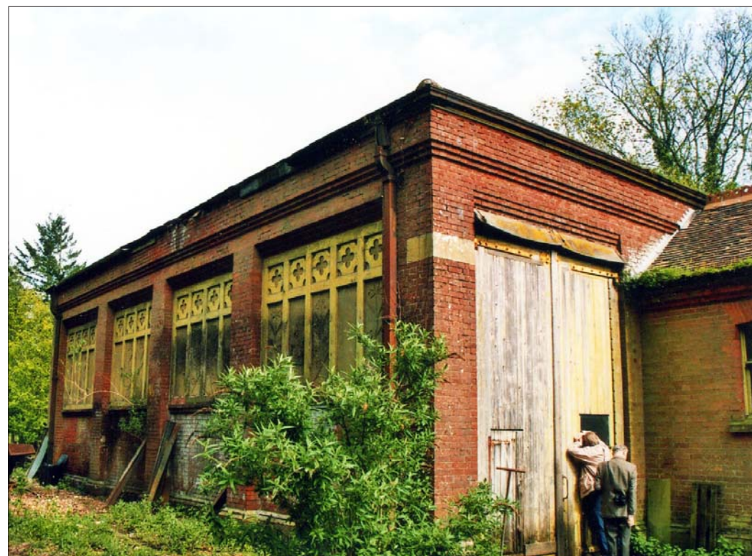
Singleton goods shed being examined by SIAS members on the occasion of the Society's visit on 3 May 2008. This shows the north (track) side of the building with the typical Myres mock-timbering and pargetting. The goods office is to the right.
