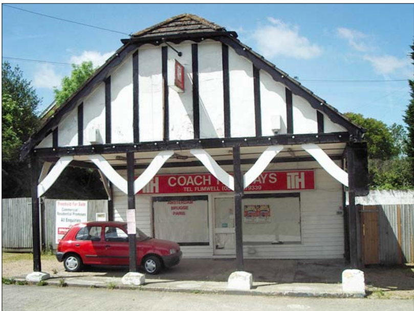
Former garage at Flimwell, Ticehurst, East Sussex. Recently listed as part of the English Heritage Cars Project. (Peter Holtham)
