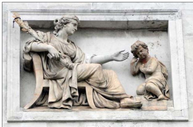
You have to look up to spot many of the Sussex examples of Coado Stone. These are on the facade of the former East Sussex County Council Offices in High Street Lewes. Now the County Court. (Martin Snow)
