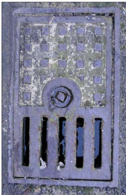
A Sewer Disconnector Cover from Margate, Kent. See the items on the mystery photo, pages 16 to 17. This example from a standard casting has the iron founders identification letters PRYK at the top left ( Martin Snow )
