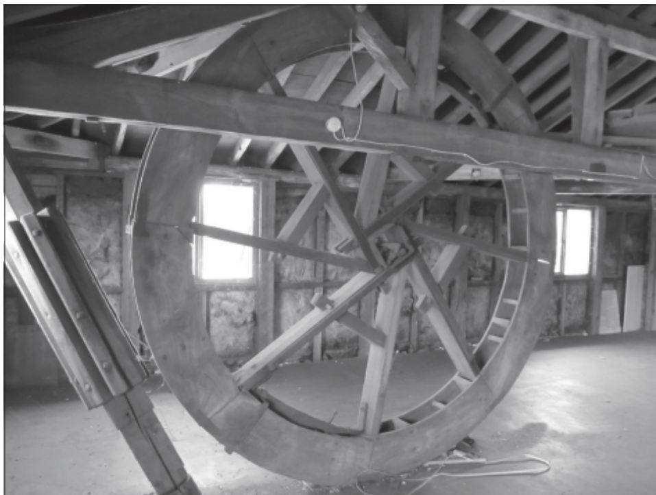
The wooden hoist wheel, removed when lift shaft was constructed. ( Ron Martin )
