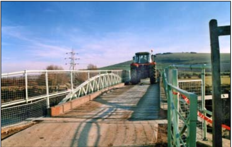
The 'first' tractor passes over the reopened Southease bridge.
