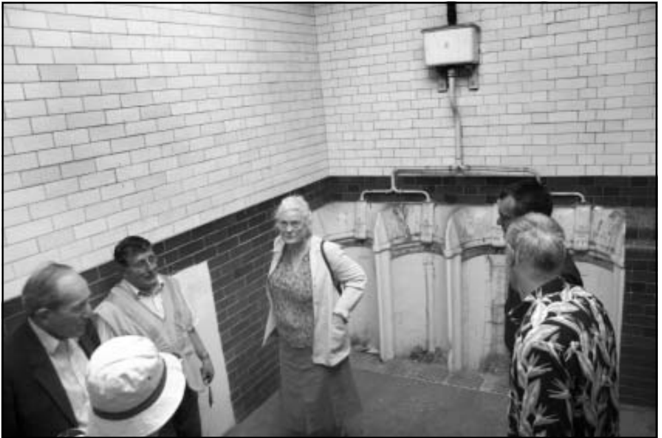
The unusual spreader system in the gent's facilities at Bexhill Central Station ( Malcolm Dawes )
