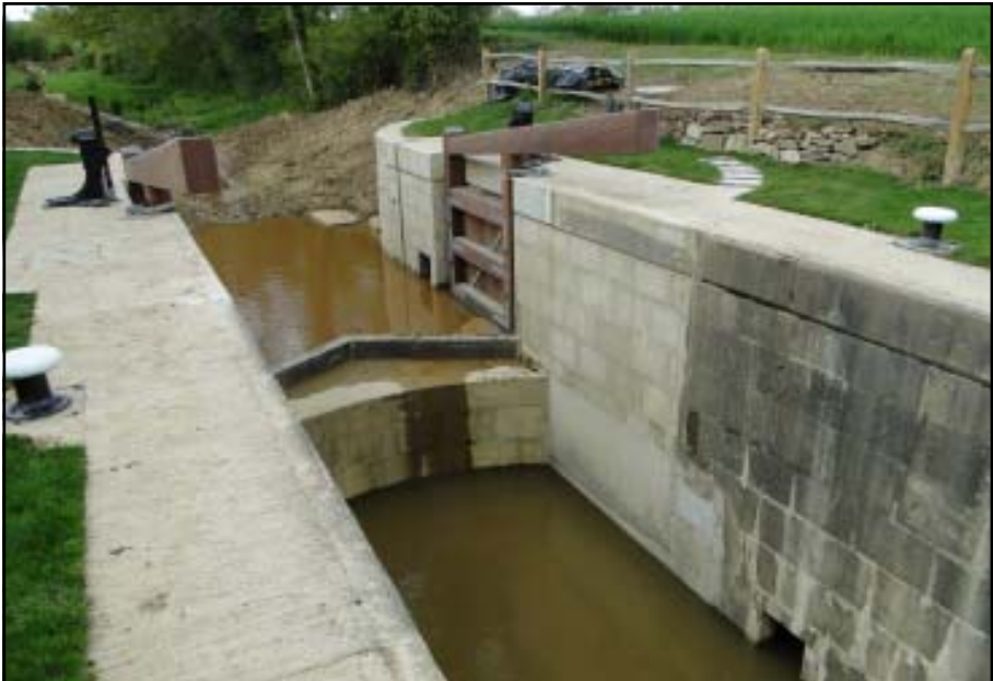
The restored Devil's Hole Lock on the Wey and Arun Canal, Loxwood. Note the lighter coloured stone of the extended lock. ( Martin Snow )
