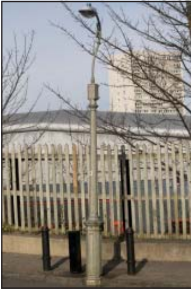
BLEECO cast iron lamp post and control box (John Blackwell)
